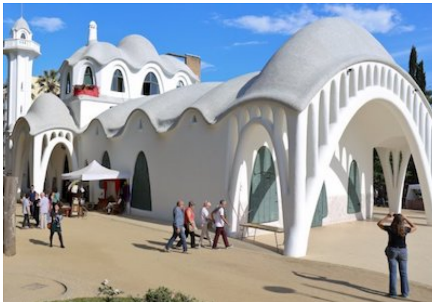
Catenary arches and Parabolic arches feature in the Gaudi inspired Masia Freixa
