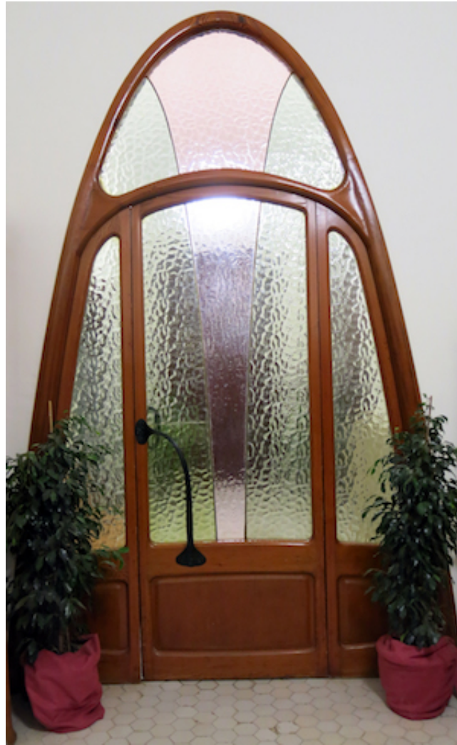
An interior door of the Masia Freixa with a catenary arched door inside a parabolic arched frame
